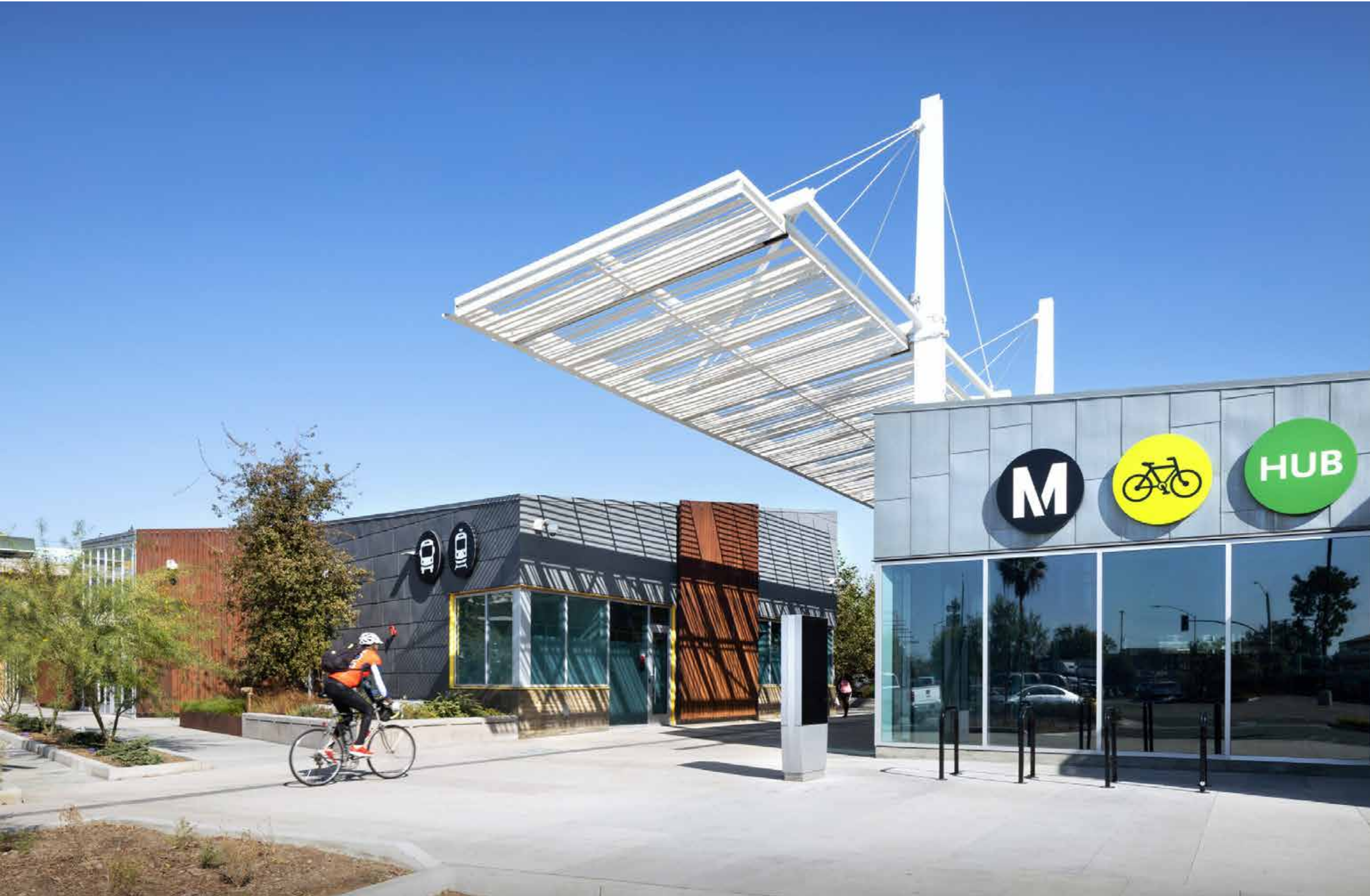
LA Metro Willowbrook/Rosa Parks Station Improvements Project Los Angeles, California, CA
