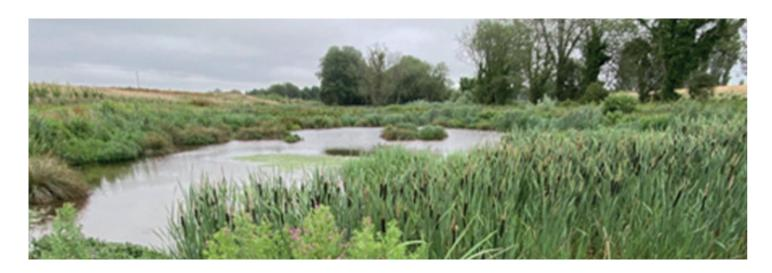
Stantec has developed the first in-catchment wetland, specifically designed to treat phosphates from surface water run off at Staplegrove, Somerset, providing a nature-based solution that would be able to offset the impacts of a 750 home residential development.
