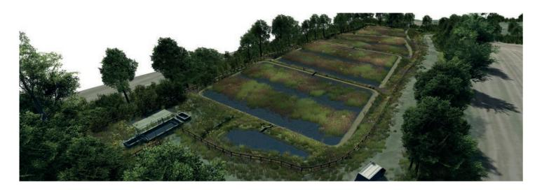
Yorkshire Water, the Environment Agency and Stantec created a Nature Based Solution (NBS) to fully replace the existing conventional treatment process, serving the village of Clifton, south Yorkshire. Clifton WwTW is located on perfect land and ground conditions to support an NBS Integrated Constructed Wetland (ICW): a low energy and environmentally friendly method of wastewater treatment -the first of its type in England treating all flows.
