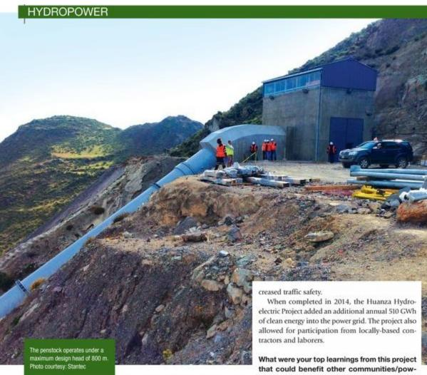
structure with a steel roof and metal cladding containing two vertical shaft generating units with a total installed capacity of 55 MVA at the generator terminals.
