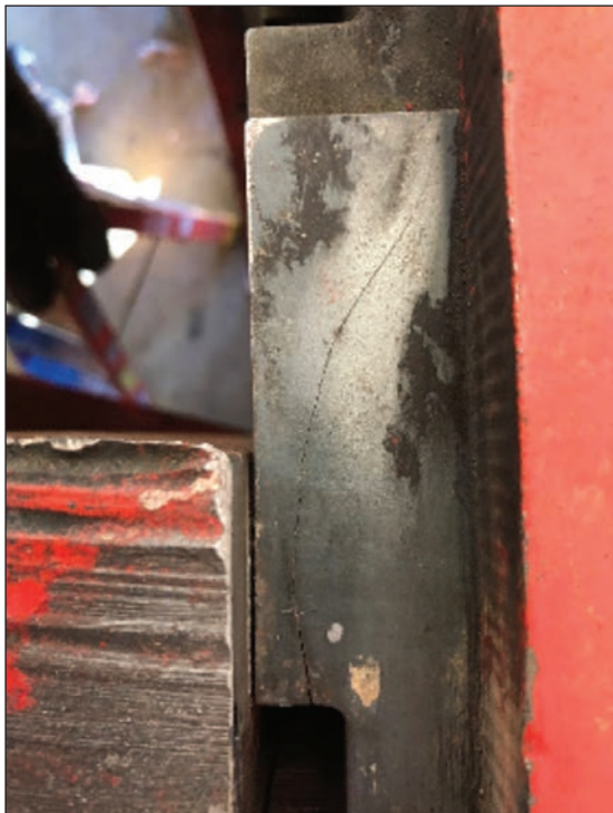
(c) Looking down on a cracked rotor rim lamination next to the shrink key slot.
