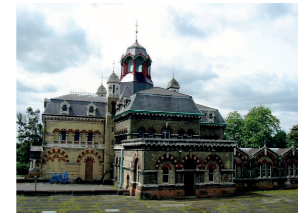
Fig 3: Abbey Mills Pumping Station. Image source: Chris Sharman
