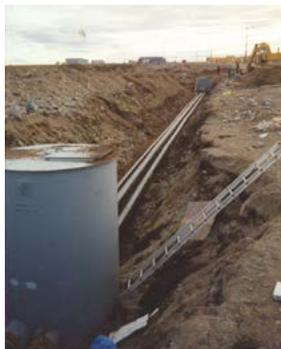
**Top:** Buried installation of insulated High Density Polyurethane (HDPE) water line in Resolute, Nunavut. **Above:** Twelve month water supply reservoir in Chesterfield Inlet, Nunavut excavated into bedrock. **Above-right:** Pump out trucked sewage collection from in house sewage tank in Repulse Bay, Nunavut. **Right:** Buried, insulated High Density Polyurethane (HDPE) water and sewer lines between manholes in Rankin Inlet, Nunavut.
