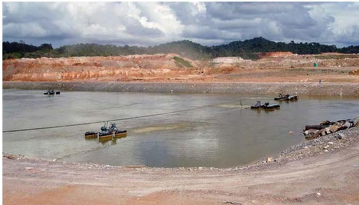
**Disadvantages:** potential limitations for filtering at the scale of this project and the large required CAPEX (both a thickener and filter press are required), higher operating costs including the cost of operating the filter plant and the added cost of conveyance and placement (either in trucks or with conveyors/stackers) and the unsaturated filtered tailings may tend toward oxidation which can result in acid generation and drainage in acid generating tailings.
