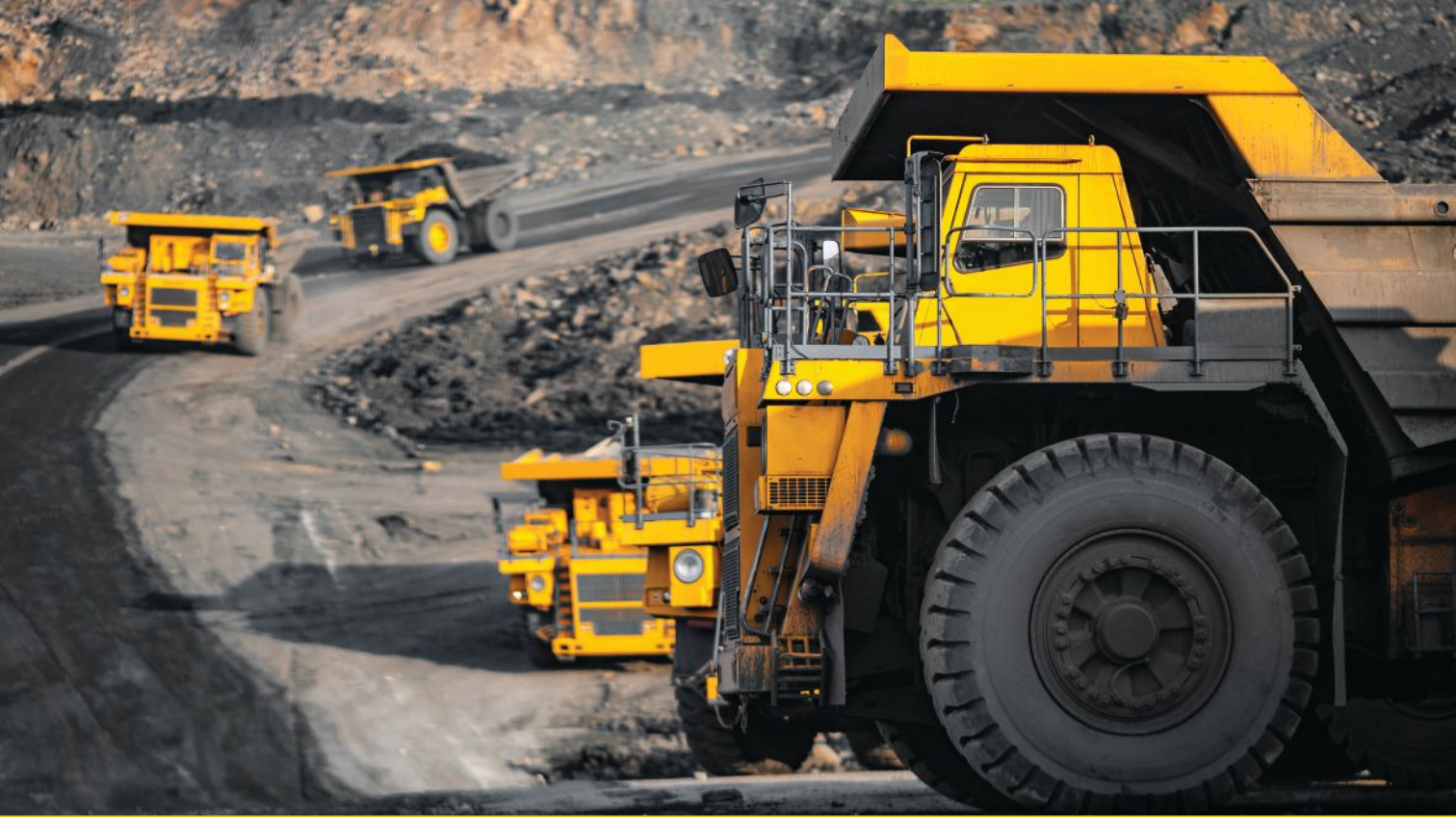
The quality of haul road plays a crucial role in the performance of a mine haulage. Photo: Stantec
