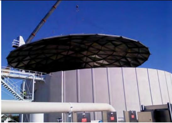
*Installation of the geodesic dome covers, June 2011*
