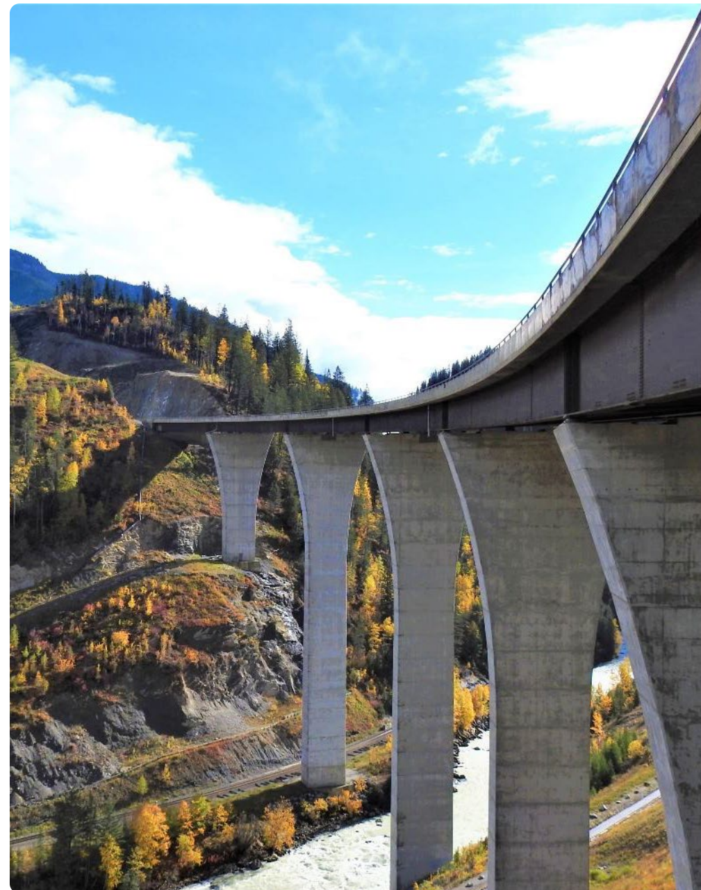
Highway 1, Kicking Horse Canyon Park Bridge Golden, BC, Canada
