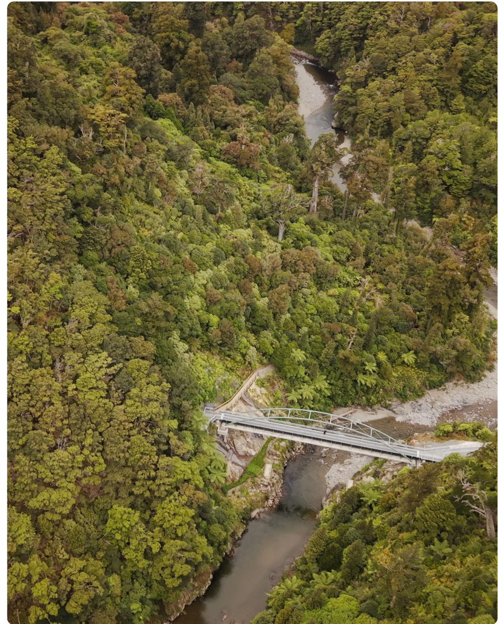
Kaitoke Flume Bridge Wellington, New Zealand
